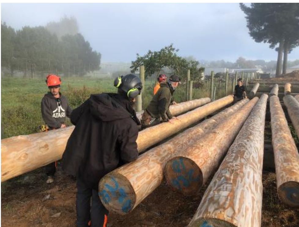
Left: Here the students are examining the debarked logs to determine the correct length, diameter and taper for their project.
